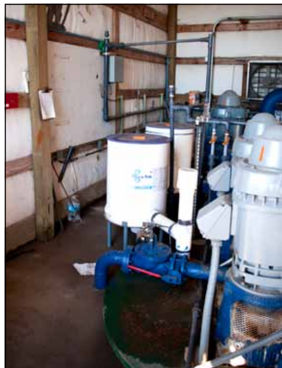
This nursery has a dedicated shed with chlorination treatment for disinfesting its irrigation water.
