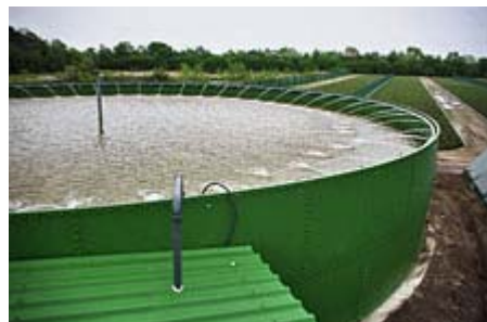
Fig. 2. Slow sand filtration (SSF) systems: (A) schematic diagram of a generic SSF system; (B) construction of the lower drainage system in an earthen basin; (C) completion of gravel layers prior to filling in an earthen basin with sand; (D) earthen basin filter during operation; (E) construction of the lower drainage system on the concrete slab floor of a steel tank; and (F) steel tank filter during operation.
