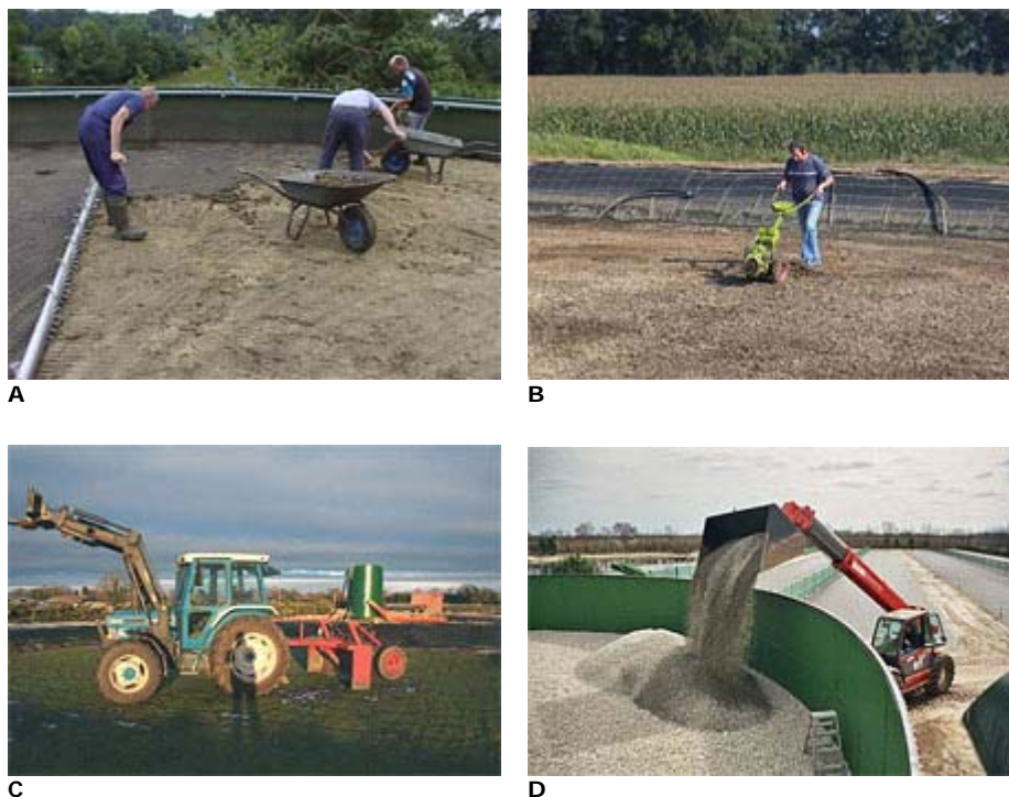
Fig. 5. Mechanical scraping and raking of the clogged layer and the re-filling of the slow sand filters: (A) manual scraping and use of a "spiny roller" (left only) to loosen layer; (B) raking with a grubber; (C) tractor with blade used to level sand surfaces; and (D) using a skid loader to fill a steel tank with filter sand.
