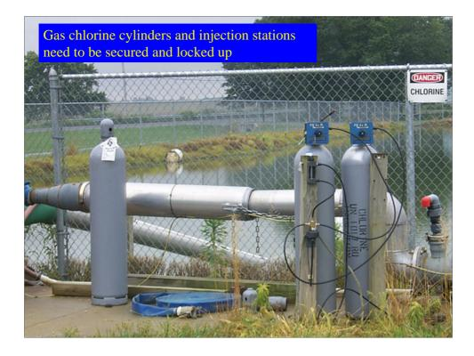
This slide represents an extremely dangerous situation since the area around the chlorination station are not secured.
