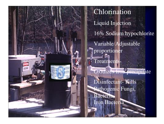
Liquid chlorine (bleach) can be injected as a disinfectant and as an oxidizer for treatment of irrigation supplies. Thorough mixing of the chlorine with the irrigation water is required for adequate disinfection.
