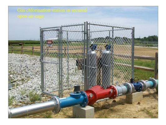
Gas chlorine is very dangerous and should be housed in a locked cage, preferably out side irrigation structures. The greatest danger occurs when gas cylinders are changed. Appropriate PPE is required for workers performing this task. This facility actually needs to be covered in an open roofed structure for best safety and protection of the injection equipment.
