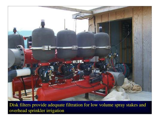
A bank of disk filters are seen in this slide. There are two banks of filters at this pumping station. Depending on the set up, one set may be filtering irrigation supplies while the other back flushes or each set may be filtering water pumped to different irrigation zones and back flushing occurs during intervals between irrigation cycles.
