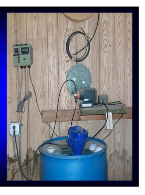
Products such as DiSolv (designed for low volume systems) or AquaSolv designed for overhead irrigation systems can be injected into water supplies as an alternative to chlorine or bromine injection. A small injection pump is use to inject low rates of these products into the irrigation system.
