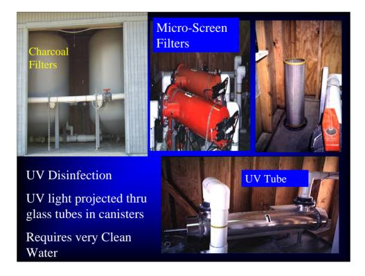
UV systems are popular for municipal waste treatment systems and can be used for disinfecting irrigation supplies. Very clean water is required for penetration of UV lamps (inside the metal covered tube-lower right picture). Lined Catch Basins and re-charging re-cycled water with fresh water supplies increases quality of irrigation supplies
