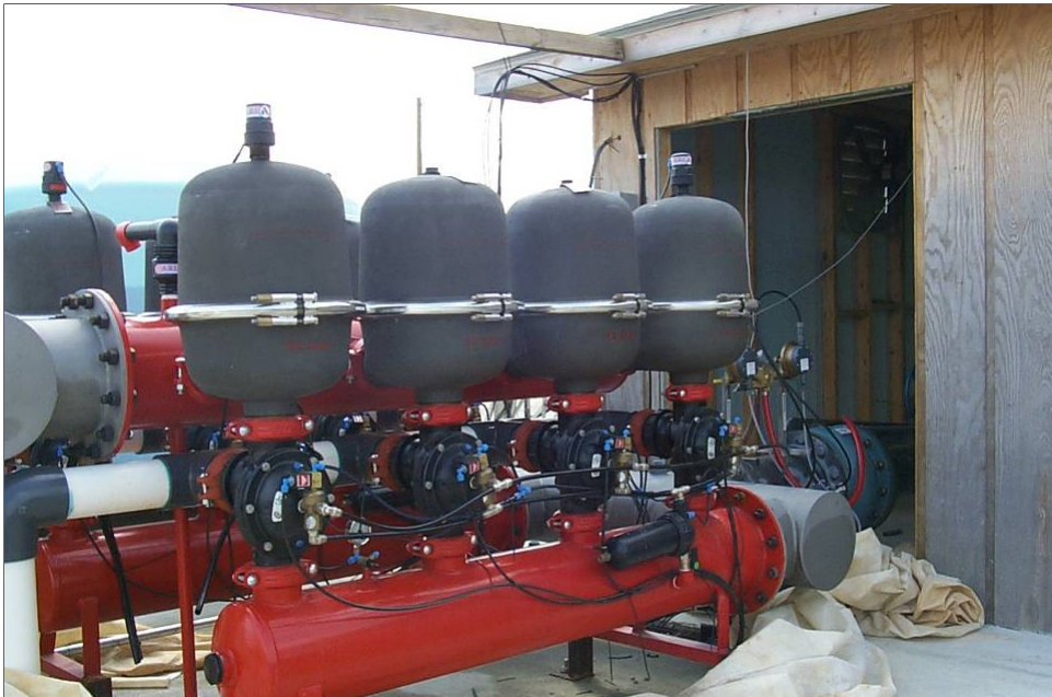
Disk filters provide adequate filtration for low volume spray stakes and overhead sprinkler irrigation
