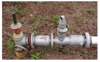
Figure 3. Backflow preventer (center) and air relief valve right.)
