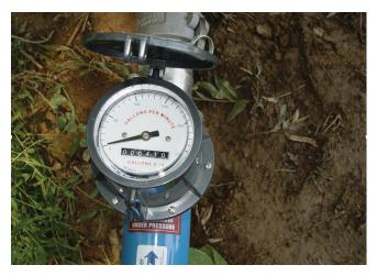
Figure 8. Flow meter for measuring the volume of water through pipes. (Photo: Anthony LeBude)
